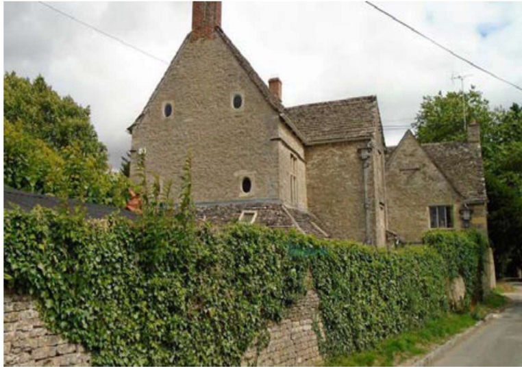
Figure 49 Roberts House. View 6C
