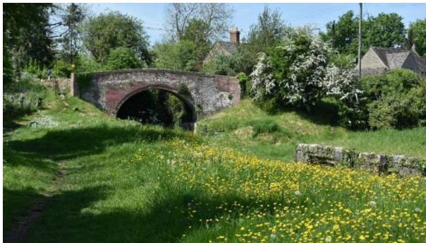
Figure 61 Upper Siddington Bridge
